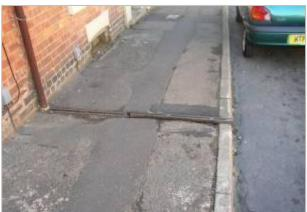
A cover, grating or frame which is higher or lower (40mm carriageways and 20mm footways) than the adjacent carriageway or footway will be classed as a safety defect. At controlled pedestrian crossing or other defined crossing points, investigatory levels will be as for the adjacent footway.
