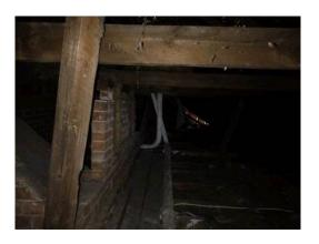
**Sample 17**: Building 135. Roof Void. Roof void. Insulation within white woven cloth to pipe running between large tanks
