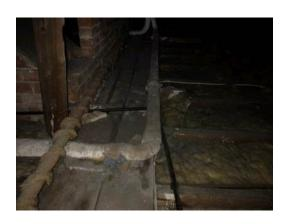
**Sample 18**: Building 135. Roof Void. Roof void. Insulation within white woven insulating pads to sides of small metal header tank
