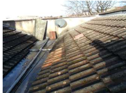
Photo: 7 Roof with Valley
