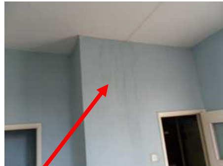
Photo: 22 Water tracking back to wall
