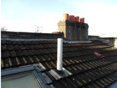
Photo: 5 Roof with Velux window
