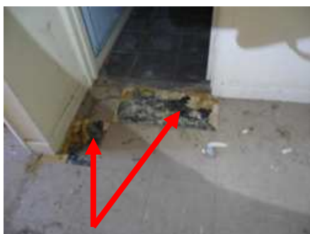
Photo: 20 Vinyl tiles removed
