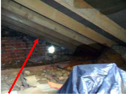
Photo: 18 Loft rafters
