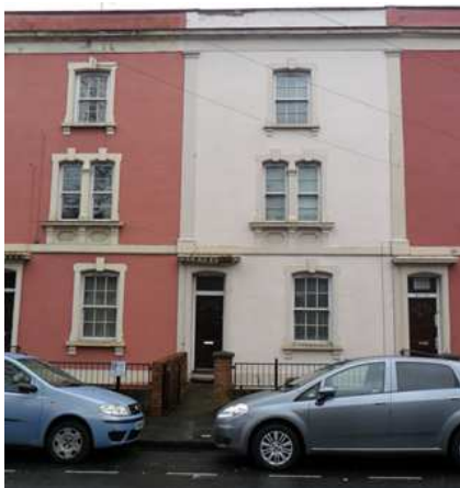
Photo: 15 No Subfloor air vent.
