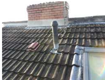
Photo: 6 Roof with new chimneystack
