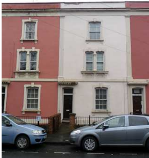
Photo: 1 Existing Front Elevation
