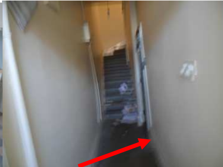
Photo: 25 slightly slanted floor
