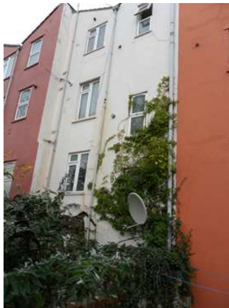
Photo: 2 Existing Rear Elevation
