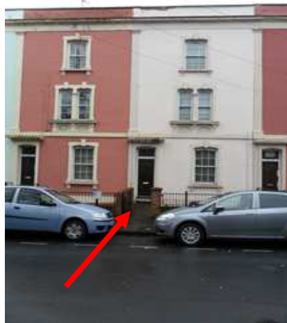
Photo: 34 Defective areas of the slab
