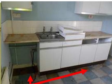
Photo: 24 Vinyl tiles removed
