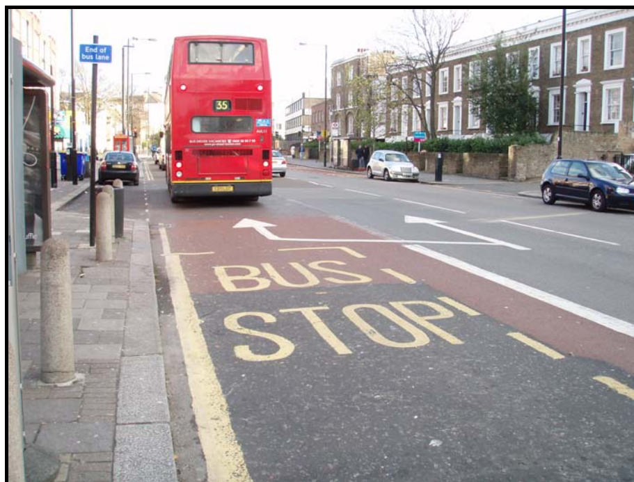
Figure 2.2 – View of the Removed Linemarking at the End of the Bus Lane
