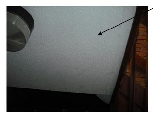
Stair Lobby 1 - textured coating to ceiling is an asbestos containing material (ACM sample BS/02). It is in good condition and recommended it be left undisturbed and monitored.
