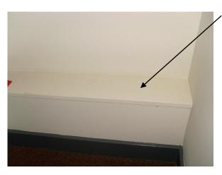
Corridor 1 - Void Behind Low Level Boxing - was not accessed (without causing damage), therefore we must presume it contains asbestos. It is recommended an inspection be carried out prior to any refurbishment work.
