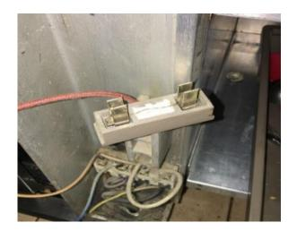
Main Kitchen – flash guard within hot cupboard 3 (identified during fixed wiring test), therefore we must presume it to contain asbestos. It is recommended an inspection take place prior to any refurbishment work.
