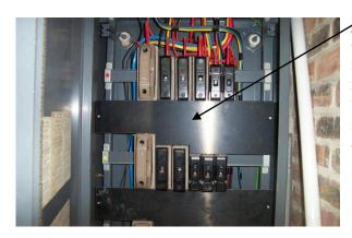
Electricity Cupboard – electrical equipment was inaccessible, therefore, we must presume it contains asbestos. It is recommended a closer inspection be undertaken prior to any invasive maintenance works. Similar electrical equipment can be found in Store 2.
