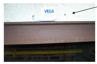
Boiler Room – panels surrounding skylight are an ACM (sample BS/16). They are in fair condition and recommended they be paint sealed as soon as possible.
