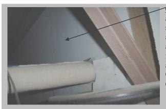
Cloakroom 1 – panel above door is an asbestos containing material (ACM as sample BS/10). It is in good condition and recommended it be left undisturbed and monitored. Similar panels can be found in the Void above Cloakroom 1, Art and Craft Room, Void above Art and Craft Room, Voids above Boys' and Girls' Toilets 1 and 2.
