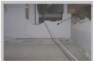
Void above Cloakroom 2 — firebreak panels above door are an ACM (as sample BS/10). They are in poor condition and recommended they be repaired and encapsulated as soon as possible. Similar panels can be found in Void above Classroom 4.
