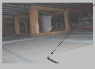
Void Above Male Staff Toilet – debris from broken skylight panels to back of ceiling is an ACM (sample As BS/04). Removal is recommended as soon as possible. Similar debris from broken skylight panels to back of ceiling can be found in the Voids Above Female Staff Toilet, Foyer, Changing Room Toilet, Classrooms 22, 25, 29, 36 and 39, Girls' and Boys' Toilet, Girls' Changing Room, and Staff Office.
