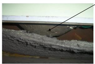
Corridor 2 – wall mounted heater, bitumen coating to motor is an asbestos containing material (ACM sample BS/02). It is in good condition and recommended it be left undisturbed and monitored. Similar wall mounted heaters can be found in the Hall, Foyer and Corridor 1.
