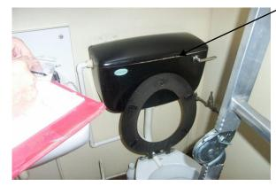
Staff Toilet—toilet cistern is an ACM (sample BS/05). It is in good condition and recommended it be left undisturbed and monitored.
