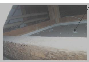
Void Above Corridor 2 – Skylight AIB debris. Removal is recommended as soon as possible.
