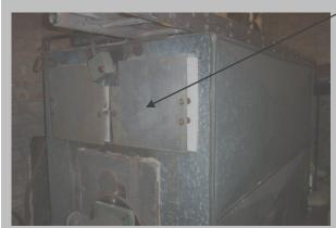
Boiler Room - boiler internal segments were inaccessible, therefore, we must presume they contain asbestos. It is recommended a closer inspection be undertaken prior to invasive maintenance works.
