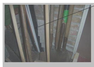
Boiler Room – redundant panel adjacent doorway is an ACM (as sample BS/18). Removal is recommended as soon as possible.
