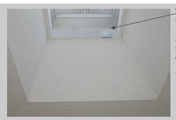
The internal strips to the skylights throughout the school are asbestos insulation board (sample BS/05). These are in good condition, paint sealed and presents no hazard to health their current condition
