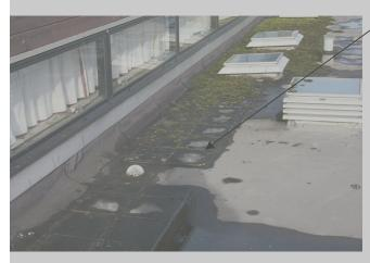
The roof tiles above the main entrance to the school are cement-based material containing asbestos (sample BS/23). These tiles are in a good condition and present no hazard to health in their current condition.
