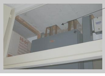
The ceiling panels in the electrical switch cupboards are asbestos insulation board (sample BS/10). These panels are in a good condition but unsealed. It is recommended that these panels be encapsulated at a convenient time with a polymeric flame retardant sealant
