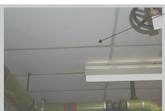
The ceiling tiles in the boiler room are asbestos insulation board (sample BS/01). These tiles are in a good condition and paint sealed. It is recommended that drilling, fixing and sanding to these tiles be prohibited.
