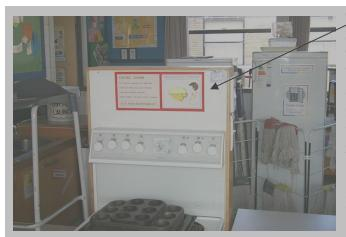
There are two cooker back panels in class 16 home craft (sample BS/11). These panels are asbestos insulation board and are generally in a good condition although some minor damage is evident in places. It is recommended that the damaged areas be repaired/encapsulated with a proprietary sealant.
