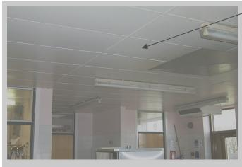
The ceiling tiles in the kitchen, kitchen office, WC, larder and vegetable store are asbestos insulation board. (sample BS/18). These tiles are in a good condition and paint sealed. It is recommend that drilling, fixing and sanding to these tiles be prohibited.
