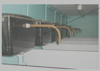
The cisterns fitted throughout the school buildings on this site contain asbestos (as sample BS/08). These cisterns are in a good condition and are unlikely to release any asbestos fibres during normal use.
