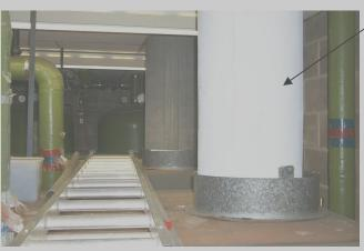
The white flue pipe in the boiler room is attached to the external flue cowl (sample BS/22). It is a cement-based material containing asbestos. This flue pipe is in a good condition and presents no hazard to health in its current condition.
