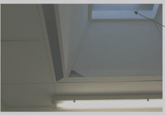
The skylight panels and skylight strips in the male and female Changing Rooms are asbestos insulation board (as samples BS05 and BS/18). These are mainly in a good condition. It is recommended that drilling, fixing and sanding to these panels be prohibited.
