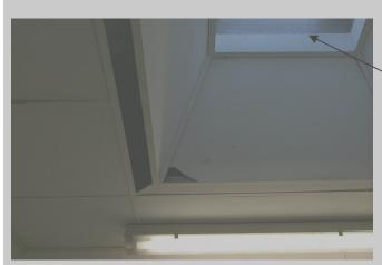
The skylight panels in the girls' and boys' Changing Rooms are asbestos insulation board (as sample BS/05). These are mainly in a good condition. It is recommended that drilling, fixing and sanding to these panels be prohibited.
