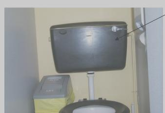
The toilet cisterns in the male and female staff toilets have an asbestos content (sample BS/08). These cisterns are in a good condition and create no hazard to health in their current condition.
