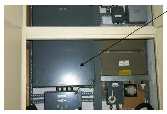
Also in the electrical switch cupboards it is strongly presumed that the electrical distribution boards may have asbestos rope material flash guards fitted to fuse holders. It is recommended that these flash guards be replaced at a convenient time with a non-asbestos product.
