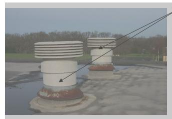
There are two flue pipe cowls on the roof of the main building. These cowls are cement-based material containing asbestos (sample BS/22). These are in a good condition and present no hazard to health in their current condition.
