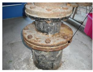
Gas Cupboard - pipe flange gaskets are an ACM (sample BS/03). They are in good condition and recommended they be left undisturbed and monitored.
