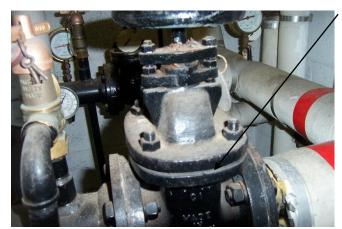
Boiler Room – gaskets to flanges are an asbestos containing material (ACM sample BS/07). They are in good condition and sealed. It is recommended they are left undisturbed and monitored.
