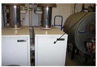
Boiler Room – boilers were inaccessible, therefore we must presume they contain asbestos. It is recommended a closer inspection be carried out prior to any invasive maintenance works.
