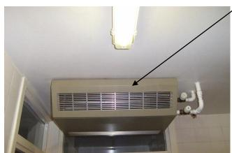
Main Area – high level wall heaters were inaccessible, therefore we must presume they contain asbestos. It is recommended a closer inspection be carried out prior to any invasive maintenance works.
