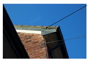
Roof – verge board strip is an ACM (sample BS/08). It is in good condition and it is recommended it be left undisturbed and monitored.
