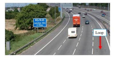
MIDAS measures the amount of time a loop is actuated by a vehicle passing over it and can therefore detects slow moving traffic.
