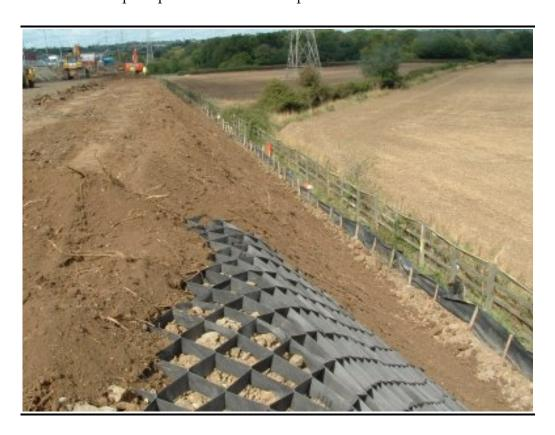
The Geocells are perforated which gives the advantage that future grass and bushes roots will grow through resulting in the artificial anti-erosion structure being woven into the roots increasing slope stability. The Geocells will be placed and nailed/anchored on the slope and filled with good topsoil. Once the topsoil has been placed, grass will be seeded on the fertile soil and for every square meter a bush will be planted. In annex xx further information is provided in relation to Geocells.
