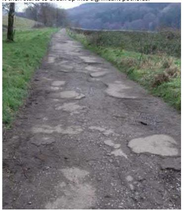
Potholed section of road = 297 5m in length, width = 3 2m with kerb stone edging, which is mostly grown over, this needs scraping back to expose the edging.
