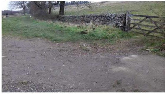
Gated barrier shown below currently comprises: dry stone wall from reservoir side, next to a small wooden stile (redundant), next to a metal vehicle gate with chain and 3 separate padlocks for different users, attached to wooden posts at either end, with a section of post and rail fencing, gas pipeline marker, adjacent to A-shaped 'squeeze barrier' to prevent trail bike usage.
