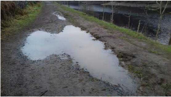
A piped culvert at 1295m is quite high beneath the current trail surface and risks overflowing, the culvert should be cleared out and the trail surface could be raised here to help prevent overspill
