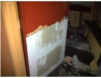
Ground Floor Kitchen highly damaged fire door with unsealed AIB lining
