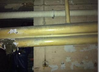
Woven pipe work insulation above non asbestos pipe work insulation in Basement Plant Room
