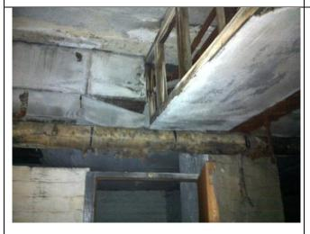
Ceiling panelling to Basement Store Room damaged to edges.
