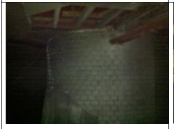
AIB Debris from damaged area of ceiling in Basement Plenum Chamber
