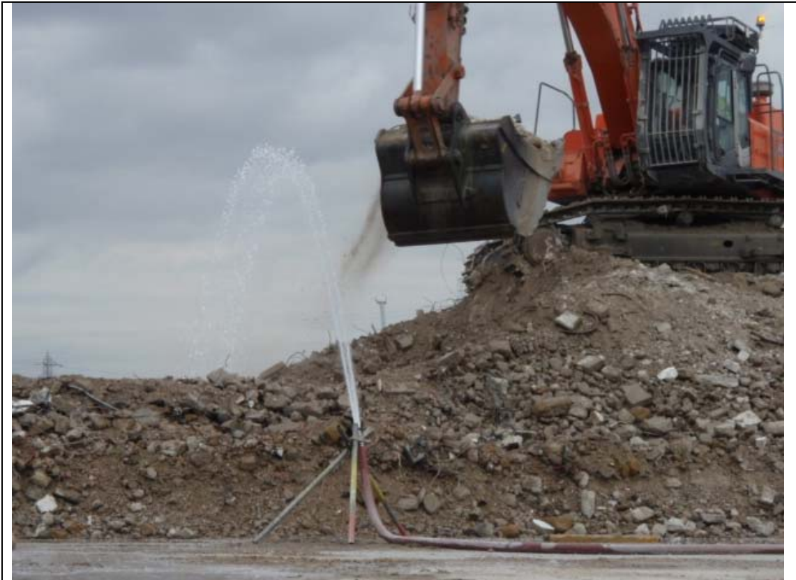
Dampening down of stockpile prior to excavation to help reduce dust
