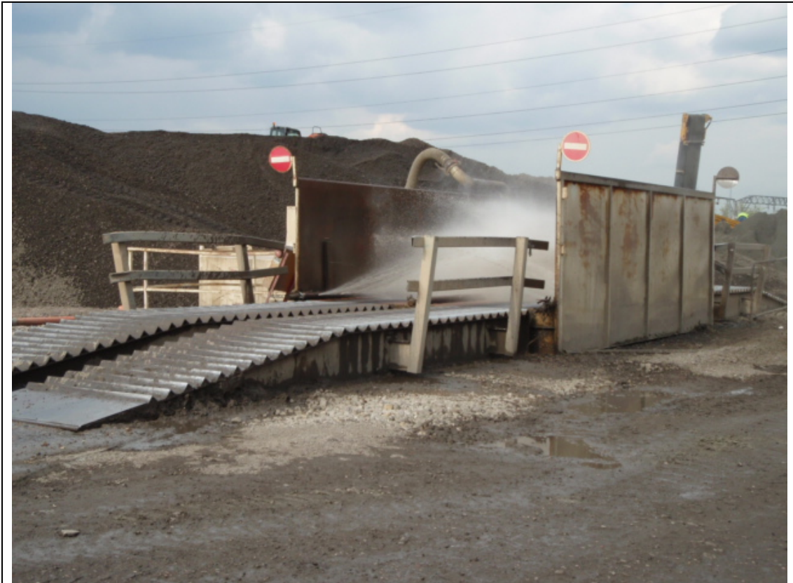
Another of the 7 wheel washes on site.
