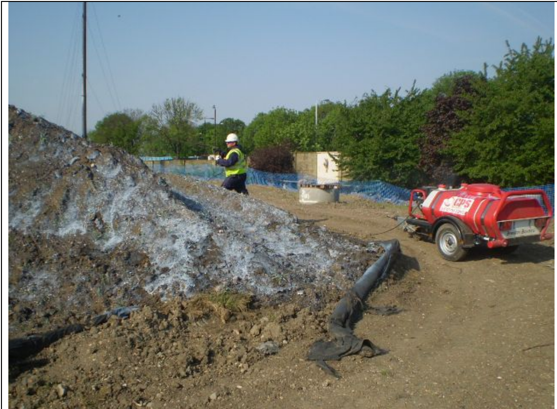
Application of Dustbuster2 onto a stockpile of material. This has been approved by Environment Agency (as it does not harm aquatic life if it enters a watercourse). This chemical binder forms a crust over the material.
