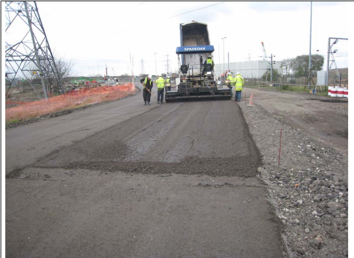
Tarmacing of new haul routes throughout site
